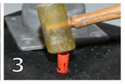
Use a rubber mallet to stuff expansion plugs into the drilled holes
