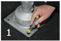
Place base plate in desired anchoring location
