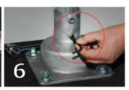
Insert post over spring, tighten both set screws to 100 ft. lbs. with a torque wrench or 3/16" allen key to hold post securely in place.
