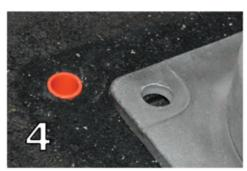
Make sure the top of each expansion plug is flush with the asphalt surface
