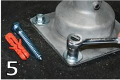
Place the base plate over the four holes and use a socket wrench with a 15/16" drive to thread all four hex lag screws
